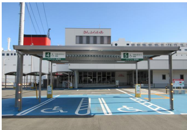
<Barrier-free parking lot>
